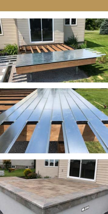
A Paverdeck Plank deck can be installed on deck pads or with frost footings. Unlike a traditional patio or deck, the steel diaphragm resists heaving and movement.
